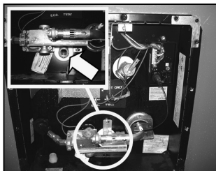
Water Heater Drain Plug Location
